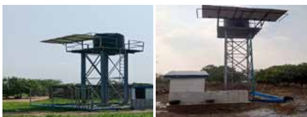
Solar-powered boreholes
